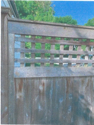
Detail of lattice at top of adjacent fence
