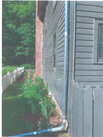
Existing gutter and downspout on house
