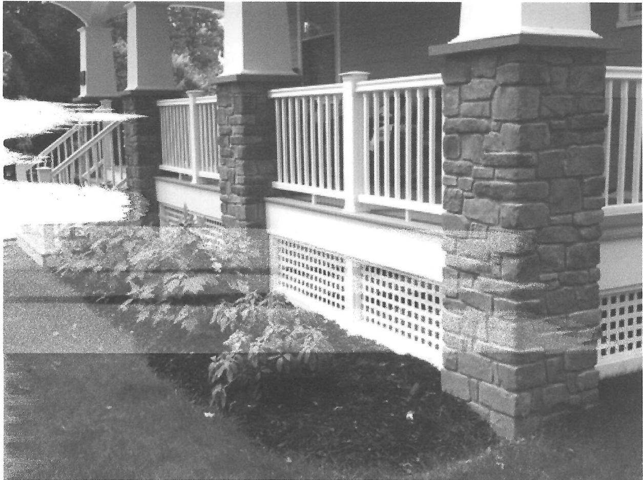
Front Porch Skirt with Square Lattice Detail Seen throughout Broad Steet
